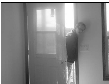
Sandy Schloss takes a peek at the interior of one of the new Staff Housing/MRHAB units.
